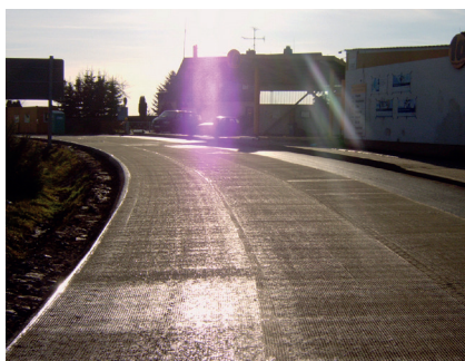
S&amp;P asfaltwapening in bochten leggen...
