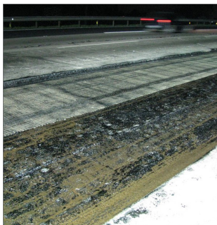
▲ S&P asphalt reinforcement grid laid onto bitumen tack coat
